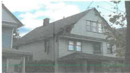
Replacing a leaking roof
