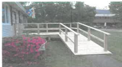
Construction of a handicap ramp
