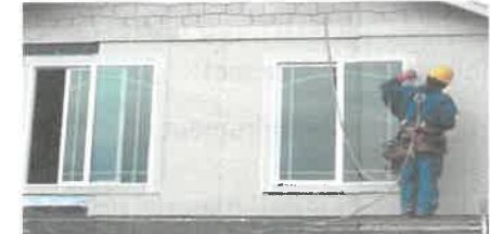
Installation of energy efficient windows
