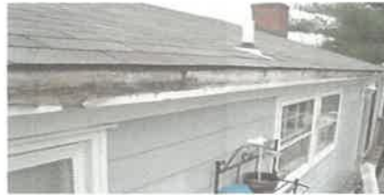
Replacement of gutters
